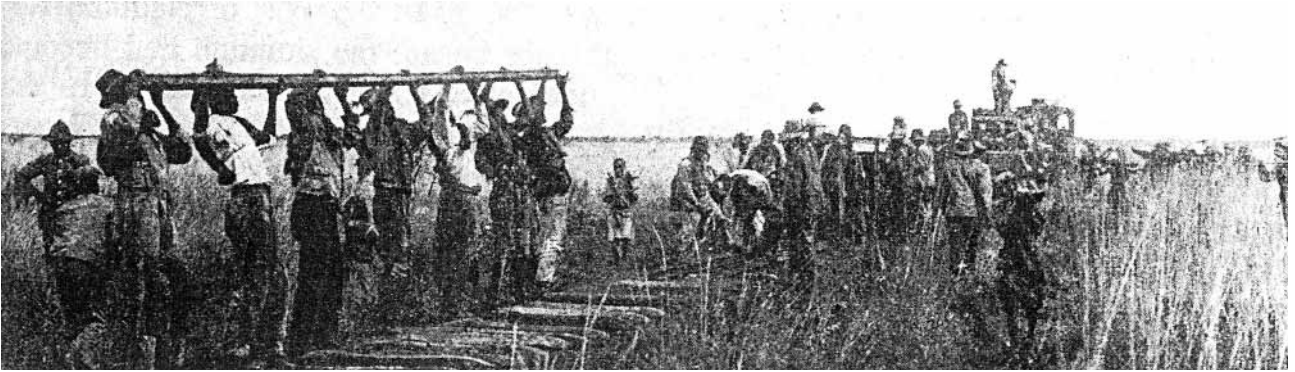
Construction of the Otavi Railway.
